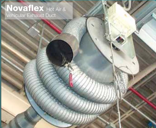
**Novaflex** Hot Air & Vehicular Exhaust Duct
